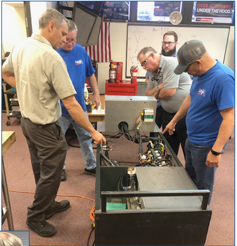
The LPIP training program is shown using the Valeo trainer in the Paratransit III HVAC class. Technicians participating in this class are Elliot Waters, Manatee, Scott Groth and Michael Erdman, Votran, and Luis Garcia, Senior Resource Association.
